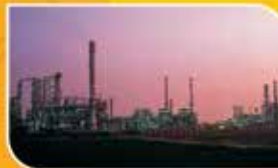
Paradip Refinery 15.0 MMTPA
